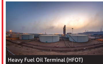
Heavy Fuel Oil Terminal (HFOT)
